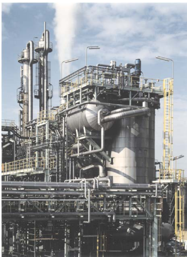
Figure 5.13. Large-scale oxo plant using the water-soluble Ruhrchemie/Rhône-Poulenc catalyst [\text{HRh}(\text{CO})(\text{TPPTS})_3] . Note the horizontal decanter in front of the reactor
