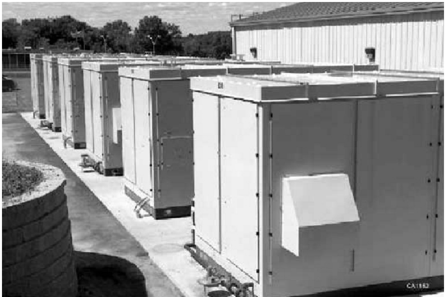
Figure 1.17(c). UTC Fuel Cells PC25 6 \times 200 kW. (Image courtesy of UTC Power Corporation.)
