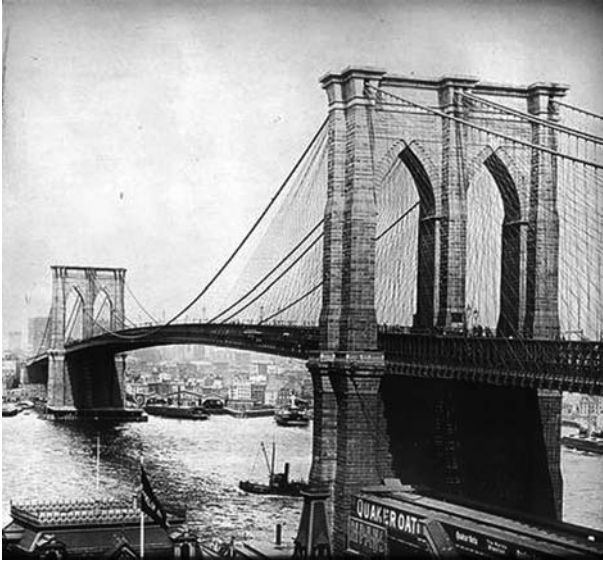
Fig. 3.12 The Brooklyn Bridge
