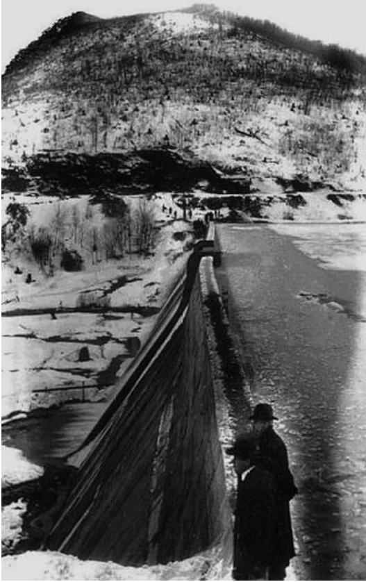
Fig. 3.18 The Austin Dam during the winter of 1910/11. Note the severe bow in the dam alignment. The two guys up front are unidentified, but one of them could well be T. Chalkley Hatton. [Photo courtesy of the Potter County Historical Society. Used with permission]
