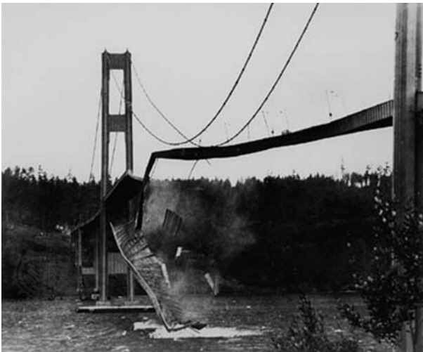
Fig. 1.1 The collapse of the first Tacoma Narrows bridge
