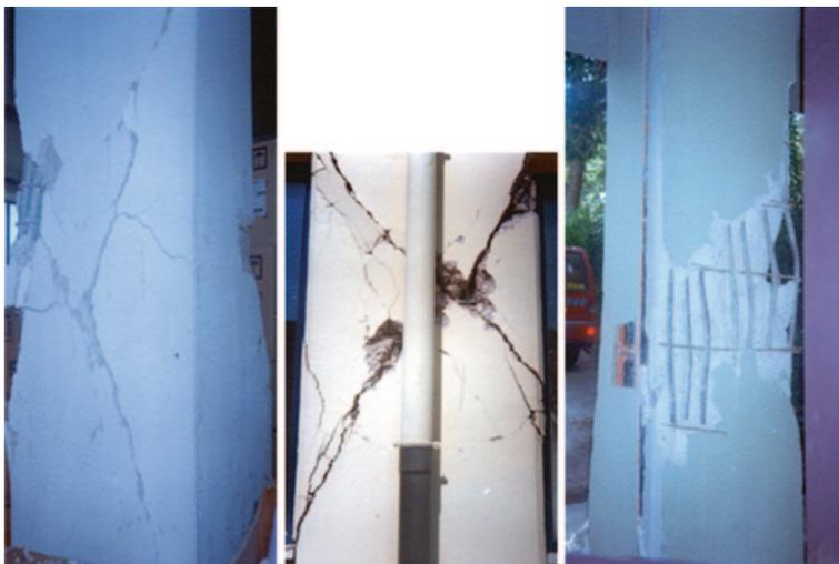
**Fig. 1.19** Examples of damage suffered by columns of RC structures during the 1999 Athens earthquake [5]
