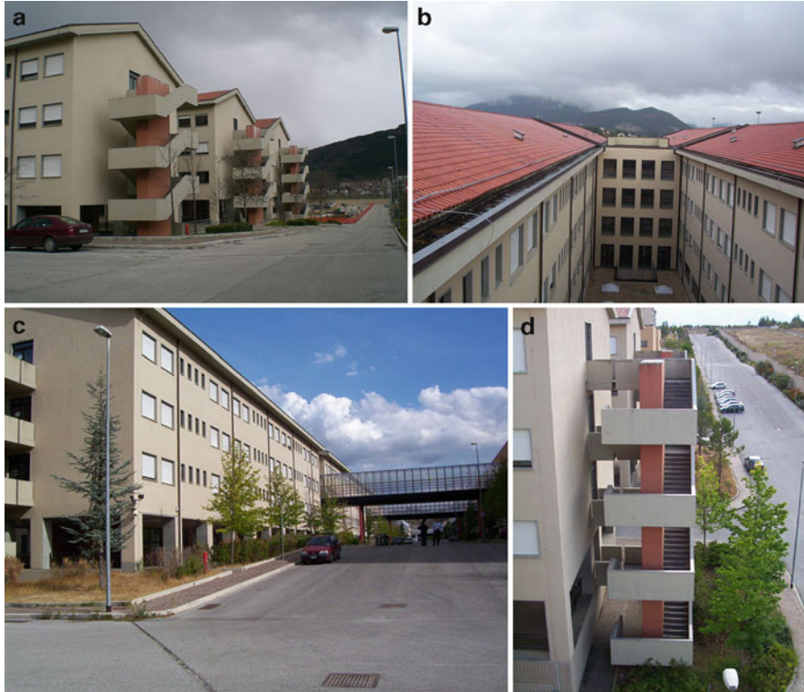
Fig. 5.15 The B1 Building Block: East side (a), courtyard (b), South side (c), outdoor stairs (d)
