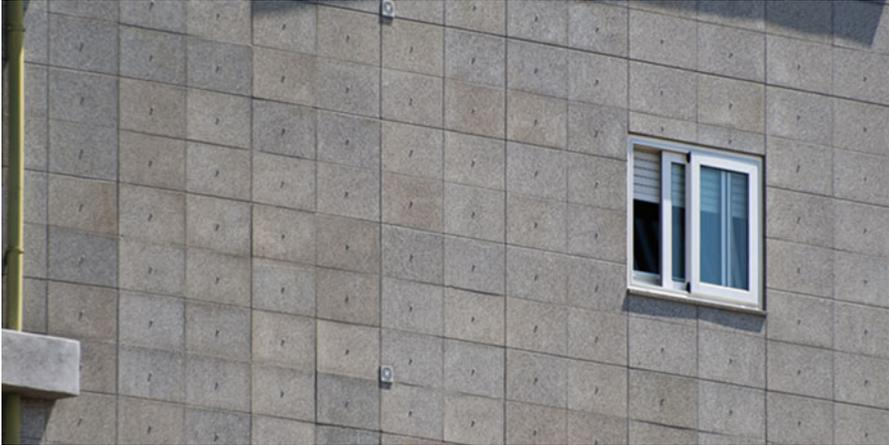
**Fig. 3.5** Façade appearance after a repair intervention with visible 8 mm screw in the centre of granite slabs previously attached with a spot bonding in a poor bedding
