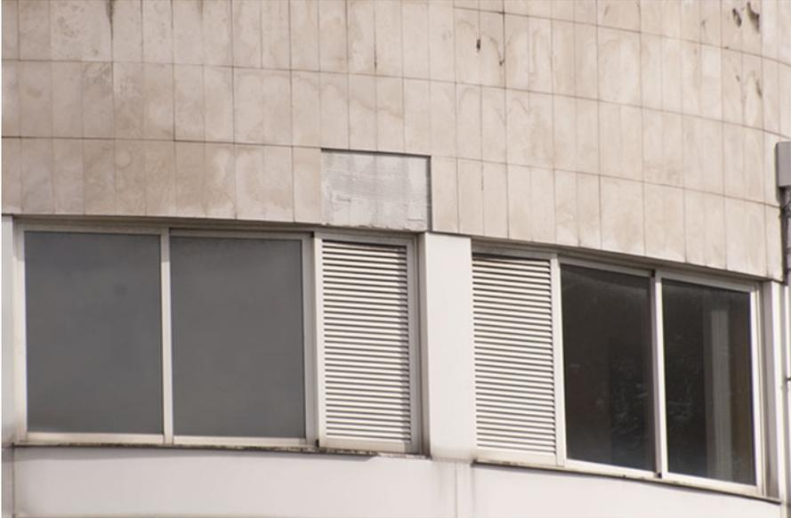
**Fig. 3.4** Cement adhered natural stone cladding detachments. *Lighter coloured* region indicates the absence of mortar in the back of the slabs symptomatic of poor bedding
