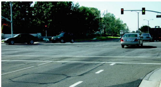
Fig. 10.22. Multiple vehicle detection loops after installation at an intersection. Courtesy of the US Traffic Corporation, Loop Application Note of 3/10/03.
