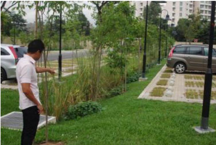
Example of a bioretention cells located in a car park
