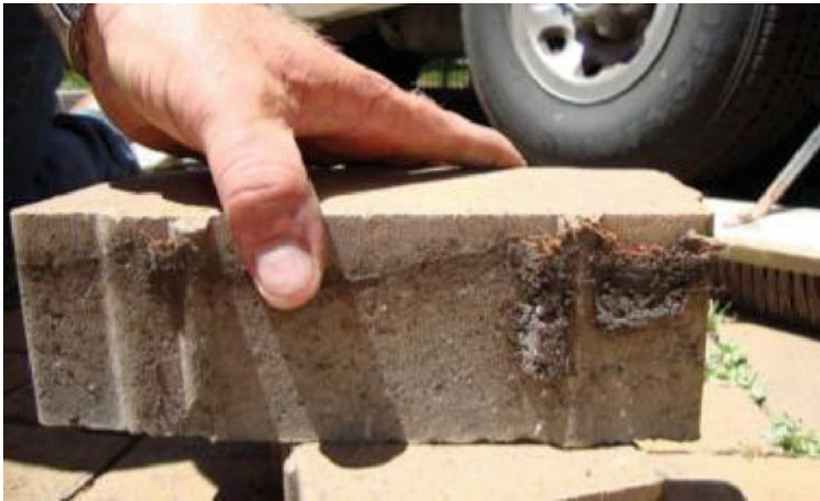
Clogged surface, or smutzdecke remnant at front of paver.
