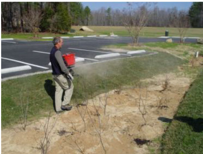
Various bioretention maintenance activities include: annual to semi-annual pruning (top), and an initial fertilization to ensure plant survival (bottom).
