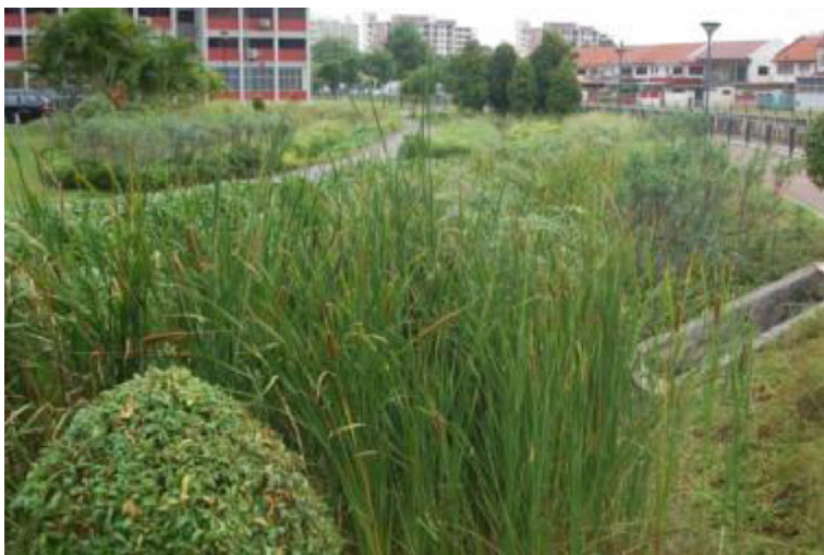
Example of a bioretention cells located in a residential community
