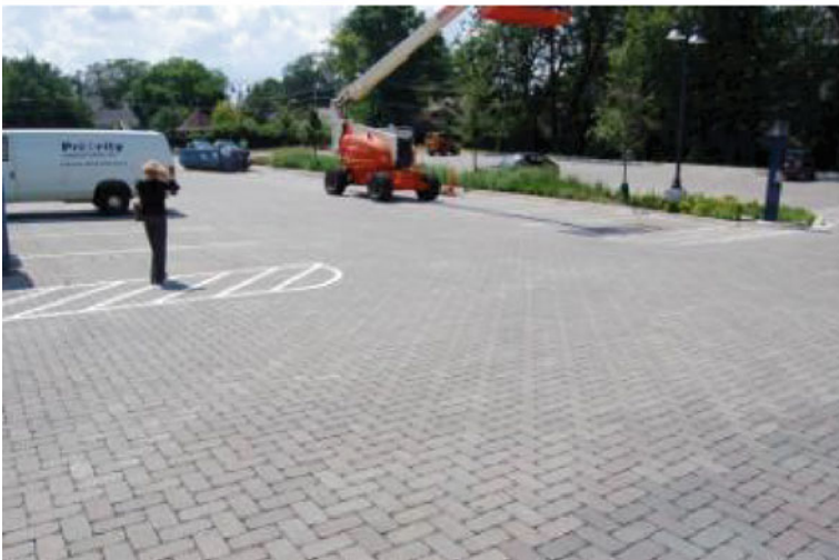
Permeable pavement installations in Singapore (top) and Illinois, USA (bottom).
