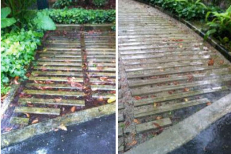
Examples of runoff occurring from “permeable” pavement
