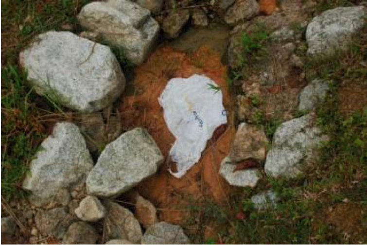
Rubbish collecting in the trough of a swale, with a modest amount of erosion.
