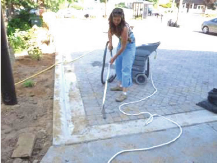
Using an industrial strength vacuum cleaner to unclog permeable pavement.
