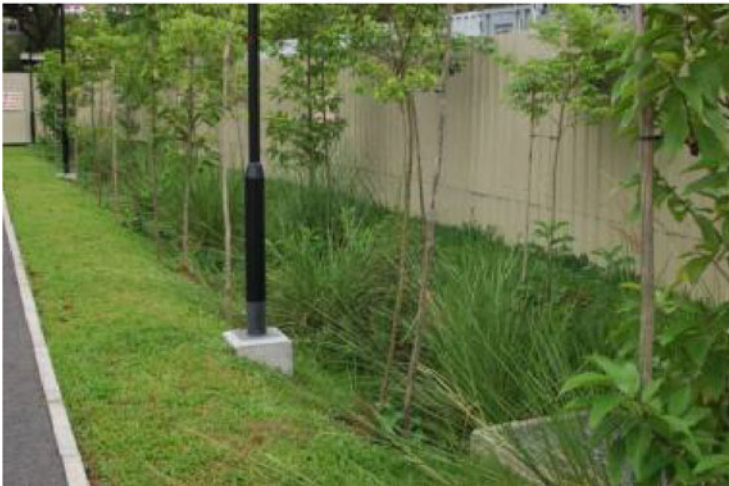
A gravel and sod verge (top) or solely a grassed filter strip (bottom) can help limit the amount of maintenance performed on the filter media in the main part of the cell.
